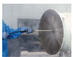
Cleaning of heat exchanger with Spin Nozzle.
